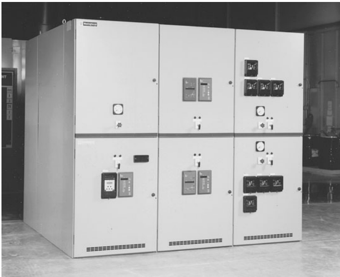
FIGURE 3.2 Medium-voltage metal-clad switchgear. (Courtesy Westinghouse Electric.)
