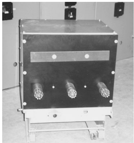
FIGURE 2.68 Rear view of a 15-kV grounding switch. (Courtesy UNO-VEN Refinery, Lemont, IL.)
